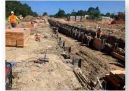
Sonoma-Marín Area Rail Transit (SMART) Windsor Rail Systems Project
