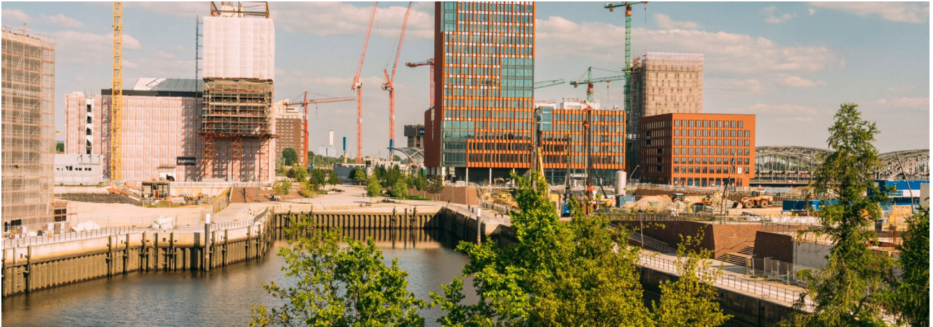
Figure 5: View of development happening in Hafencity. Note elevation of area above water level (Miguel Ferraz, hafencity.com).
