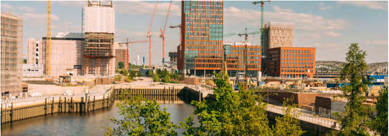
Figure 5: View of development happening in Hafencity. Note elevation of area above water level (Miguel Ferraz, hafencity.com).
